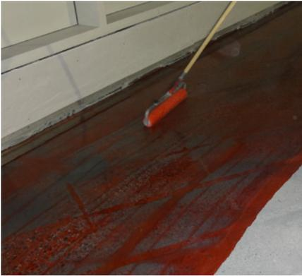
Moisture mitigation was followed by application of TechPrime™ A Advanced Acrylic Multi-Surface Primer. TechPrime A prepares both porous and non-porous surfaces for the application of any CustomTech self-leveling underlayment and improves the bond to the subsurface. This solvent-free formula was roller-applied directly over the dried TechMVC. TechPrime A dries in as little as an hour to receive leveler and speed fast-track installations like airports.
