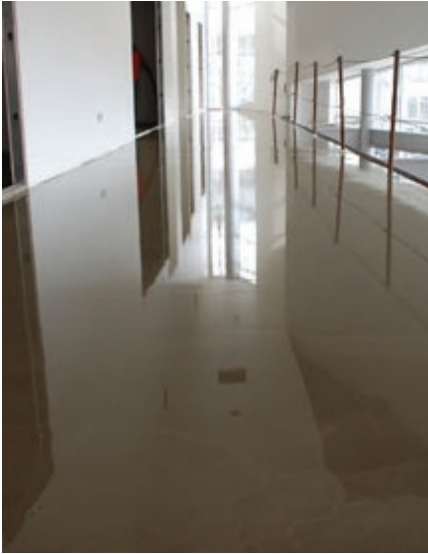
Photo Courtesy ABW Construction – Woodinville, WA
